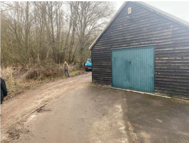
6. Looking North with the driveway curving behind the timber building..
