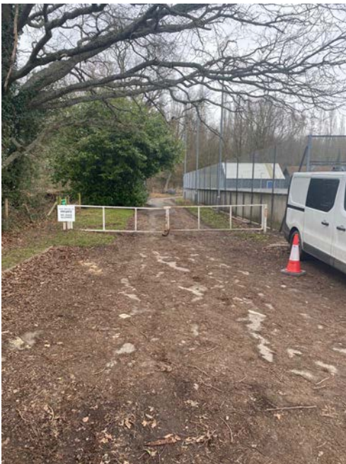
4 . Lightweight steel gates adjacent to van parking.
